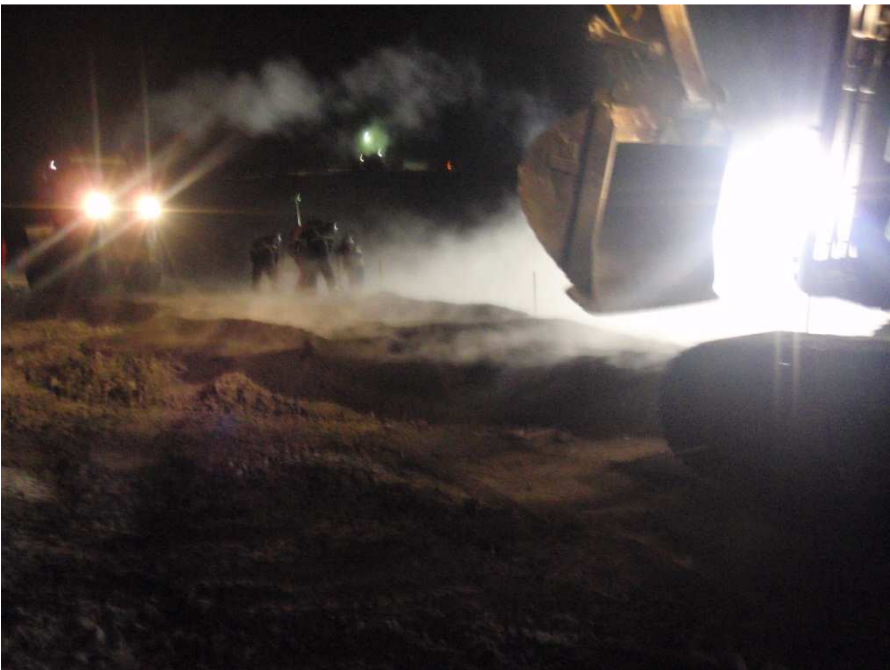
Photo 12: Excavator spreading FCM and labourers sloping side slope.
