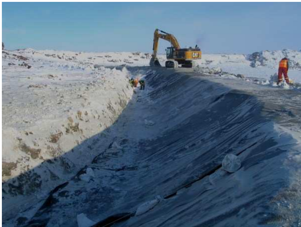
Photo 10: Preparing for overliner bentonite around Stn 3+30 to Stn 4+45 at the berm
