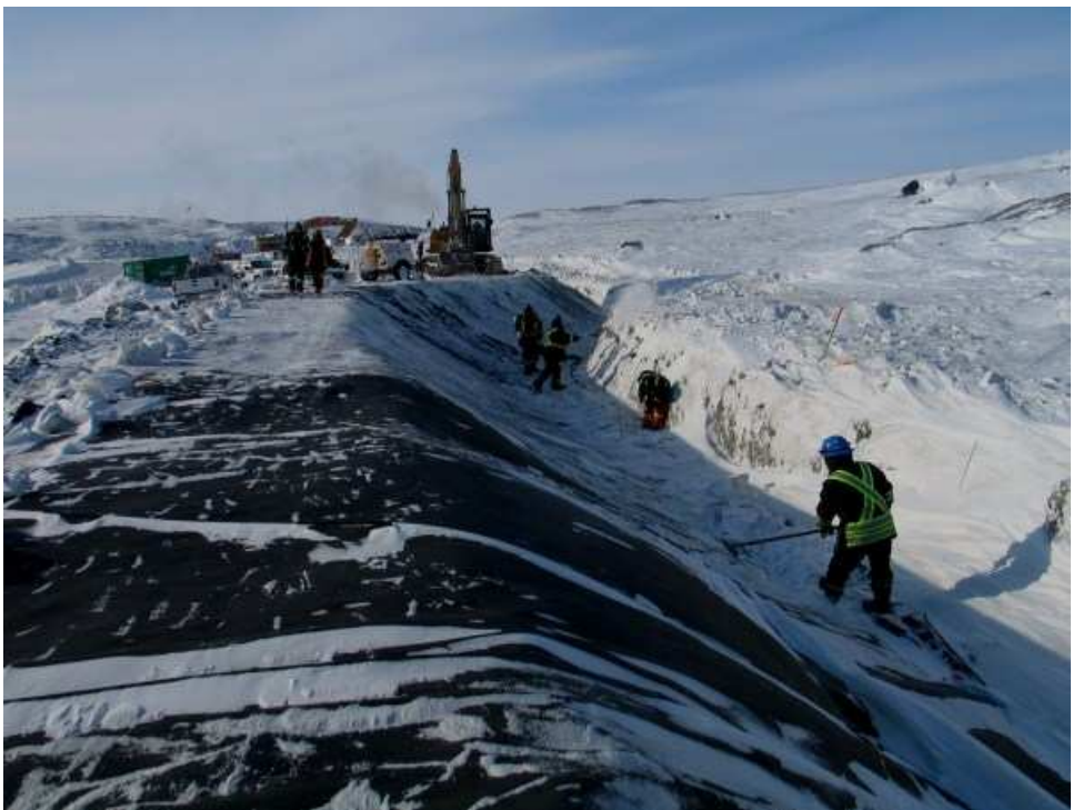
Photo 9: Cleaning snow off geotextile Stn 3+30 to Stn 4+45 at the berm
