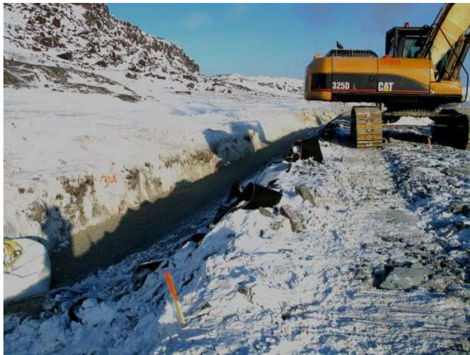
Photo 7: Bentonite placed Sta 2+95 to Sta 3+30 at the berm
