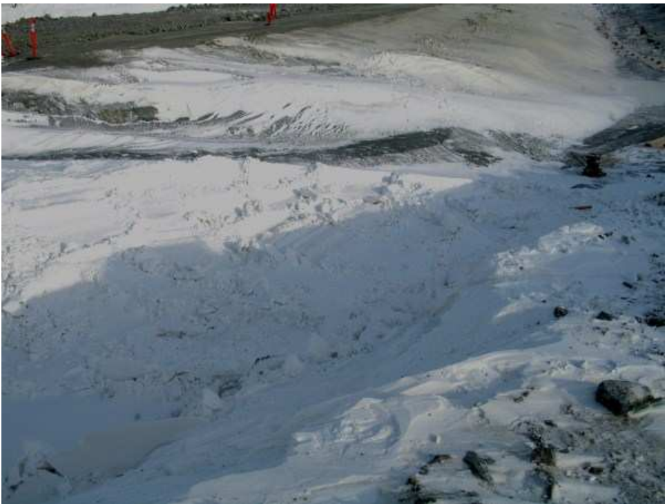
Photo 4: Some snow clearing over GCL at south end of core.
